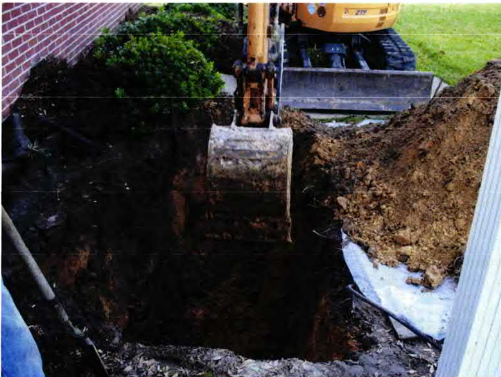
Picture 2: UST 413Elderberry excavation in progress.
